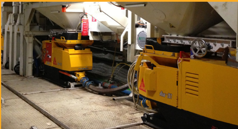
Pea gravel backfilling installation on TBM
