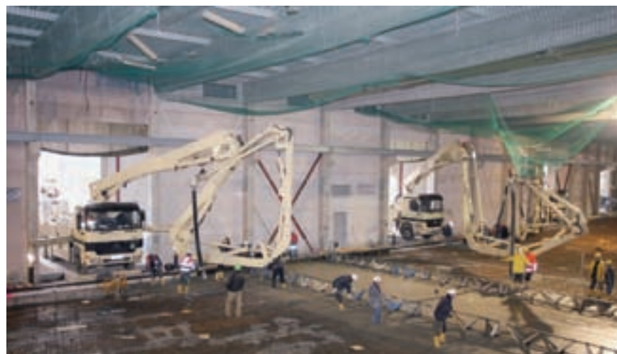
Thanks to the minimal unfolding height of only 5.7 m, the M 31-5 is unbeatable for hall concreting
