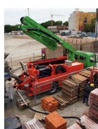
The flexible Z roll and fold 4-arm boom is able to access the smallest of openings in a building without the slightest effort. With hose extensions – attached to the boom end or directly onto the hopper outlet – the M 20-4 is the master of renovation work. (Illustrations show some optional equipment.)
